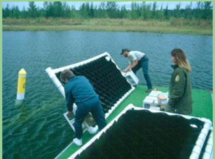
Artificial fish attractors require more time and money to construct, but are just as effective as brush attractors and last almost indefinitely.
